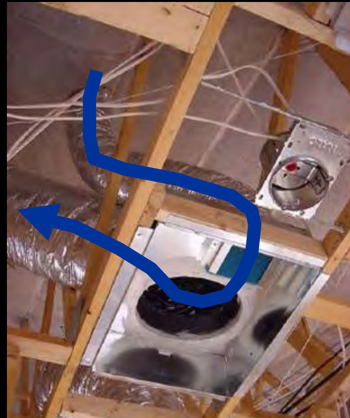
DUCTED FRESH AIR SUPPLY
