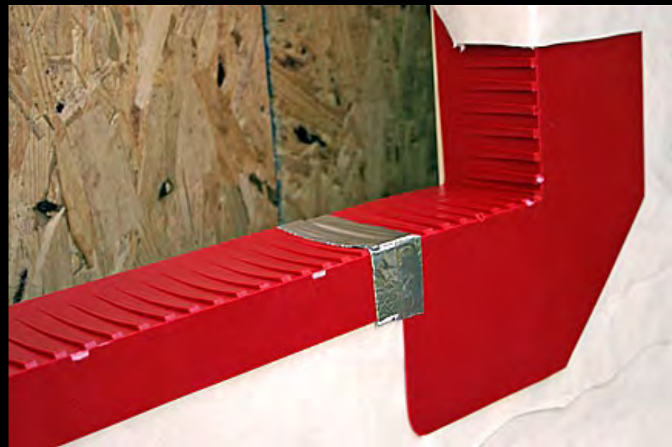
WINDOW/DOOR PAN FLASHING
