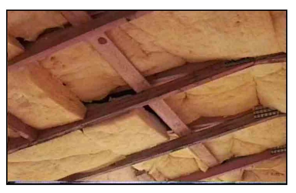
2. *Ceiling insulation*performance is dependant on a continuous air barrier.
