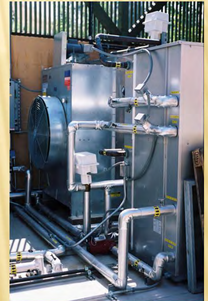
Absorption Chiller and Cooling Tower
