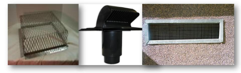
Corrosion-proof rodent/bird screens for openings (e.g., copper or stainless steel mesh) <u>Exception</u>: clothes dryer vent
